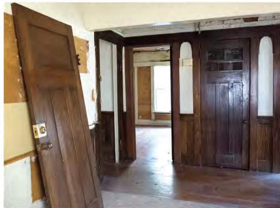
The upstairs hallway with a view to a bedroom, the woodwork with Stickley's distinctive corbels.
