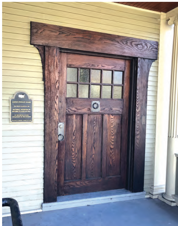
Framing and corbels surround the front door to Stickley's home.
