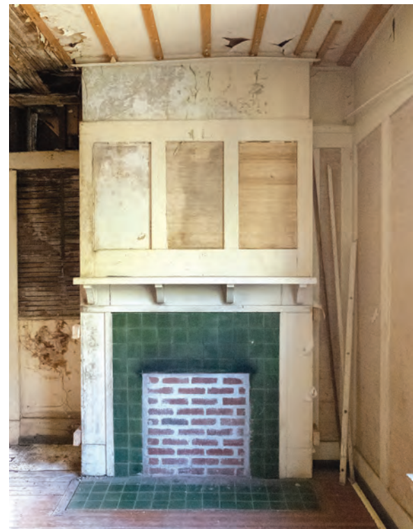
A second-floor bedroom with a fireplace surrounded four-inch square mat green Grueby tiles.
