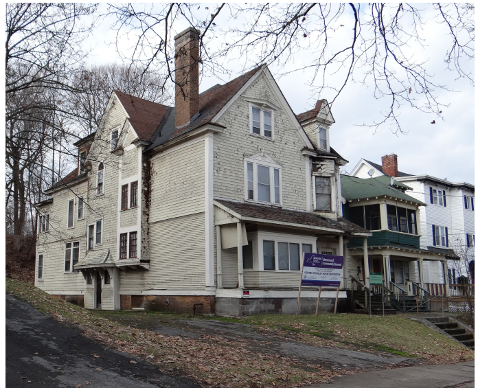
Exterior of Gustav Stickley House, prior to February 2017
