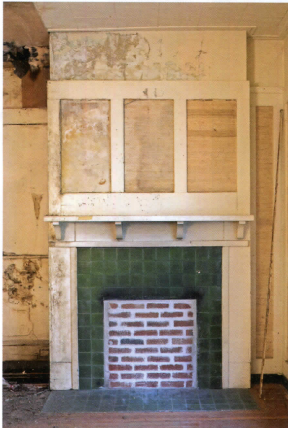
TOP, A PAINT CONSERVATOR TAKES SAMPLES FROM THE EXTERIOR OF THE HOUSE. BOTTOM, A FIREPLACE IN A SECOND FLOOR BEDROOM IS SURROUNDED BY GRUEBY FAIENCE TILES.
